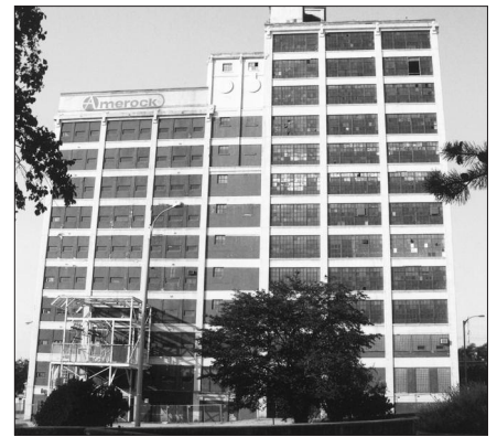
Ziock Building, Rockford
