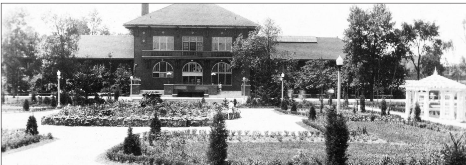
Hatzfeld's original design for Independence Park included this field house with an adjacent ball field. Ball players often broke windows in the field house, so park officials asked Hatzfeld to modify the landscape design. He replaced the field with a garden, fish pond, pergolas, trees, and shrubs. (Photo courtesy Sandy Altman)
