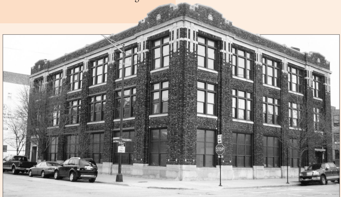
Creamery Package Manufacturing Company Building, Chicago
